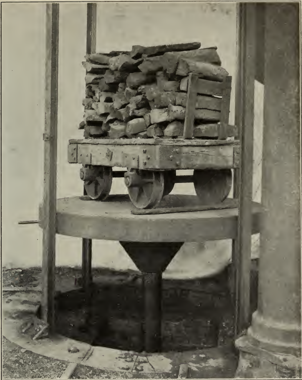
HYDRAULIC CUPOLA HOIST, R. D. WOOD & CO., PHILADELPHIA.
